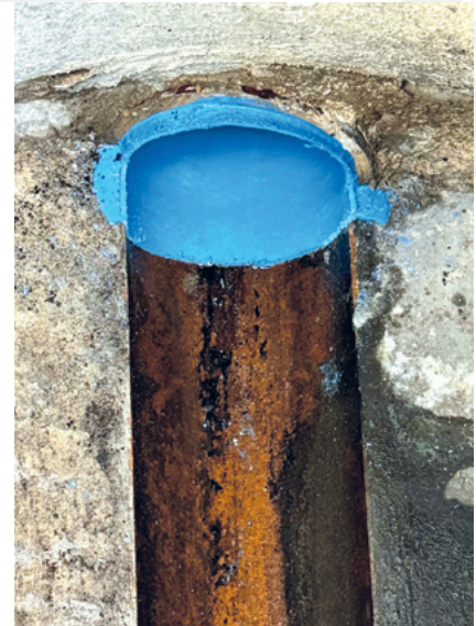
Base pipe after renovation
