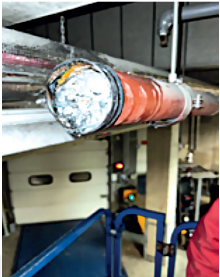
Underdrain pipe total blockage
