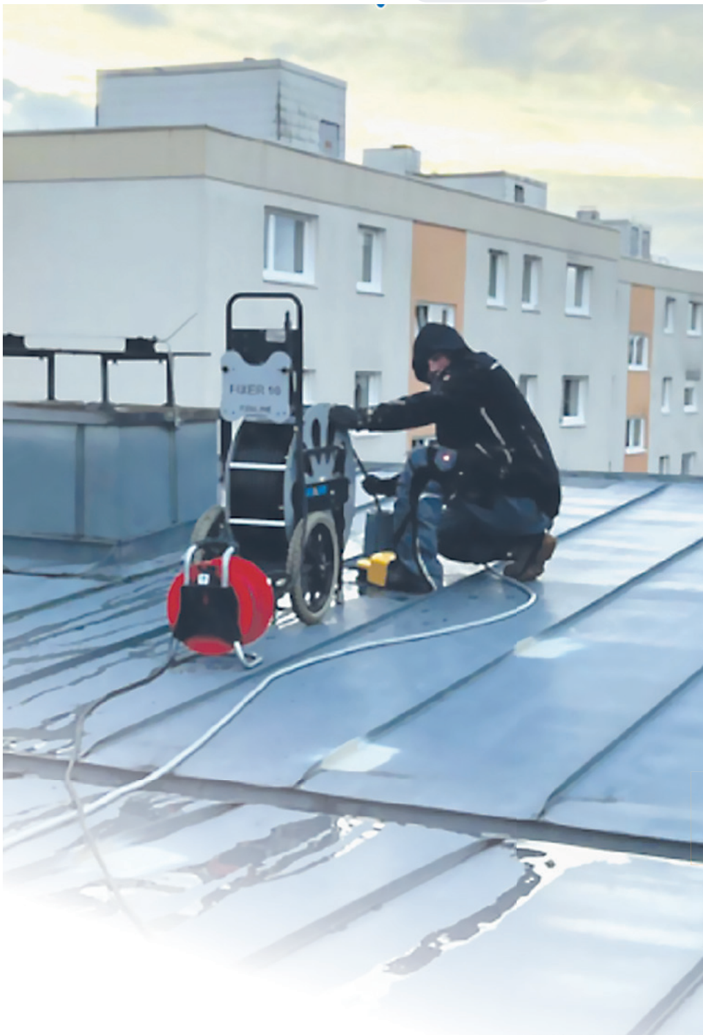
Milling work on a downpipe starting from the flat roof
