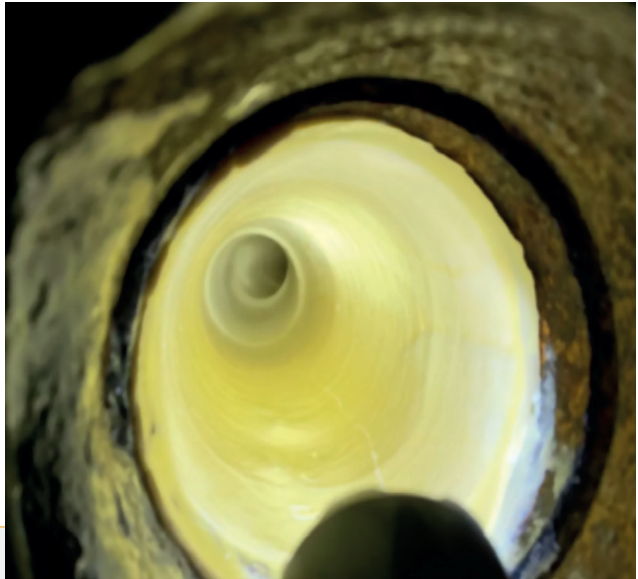
Repair of a main line using the point liner system
